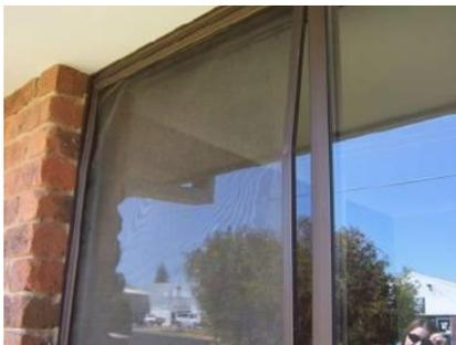
This flyscreen frame was damaged when the tenant had locked their keys inside and tried to take off the screen from the outside to get through the window!
