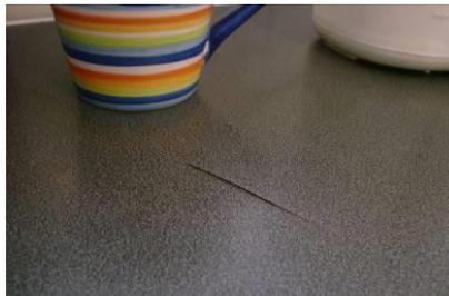
Unfortunately this separating join in the bench-top will greatly worsen over time due to swelling chipboard affected by moisture underneath!
